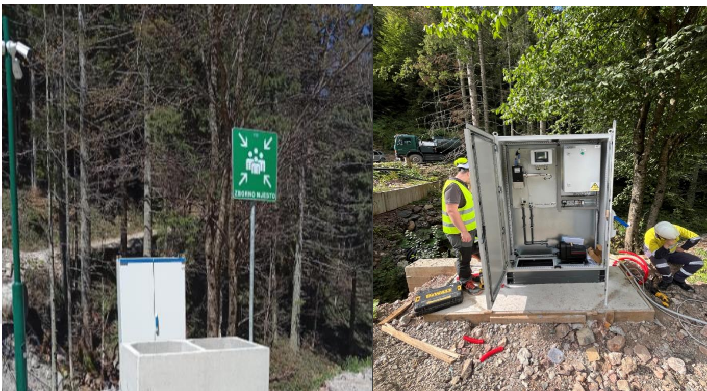
Picture 3. Installation online monitoring station (Vrući potok)
